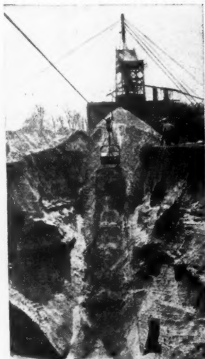
Sauerman Slackline Working In Dry Deposit.
